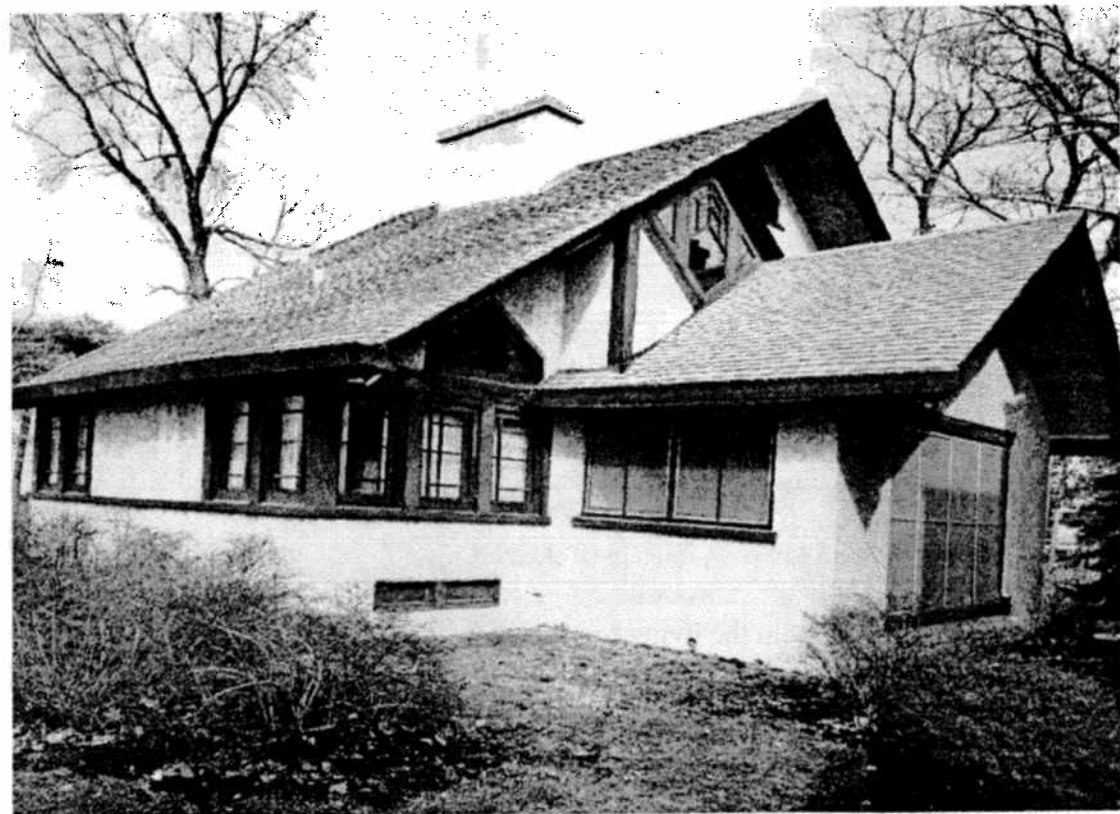
Top: Striking corner window groupings (with unusual fixed transom panels above) of the Peters House are characteristic of its Prairie style detailing. Bottom: The front (west) elevation of the house.
